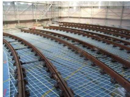
Floor slab Tram Depot Basel, CH 2009
